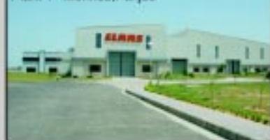
Plant 1 - Morinda, Punjab
