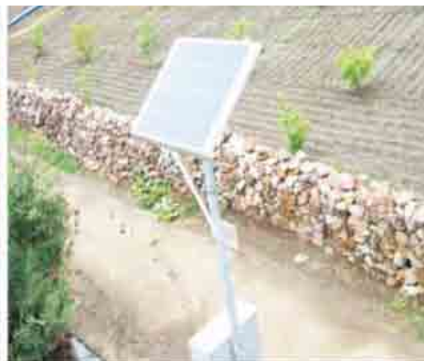
2. Solar lights Installation during 2nd Visit
